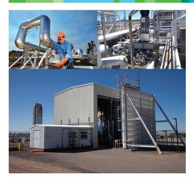
concentrated flux sequentially to expose the samples to predetermined temperatures, fluxes, and/or durations. The peak irradiance is ~1.1 MW/m² with an average irradiance of ~0.9 MW/m² over a spot size of ~1 inch (2.5 cm).
