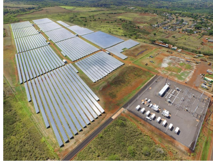
Saft 6 MW / 4.2 MWh ESS Kauai - Grid Stability
