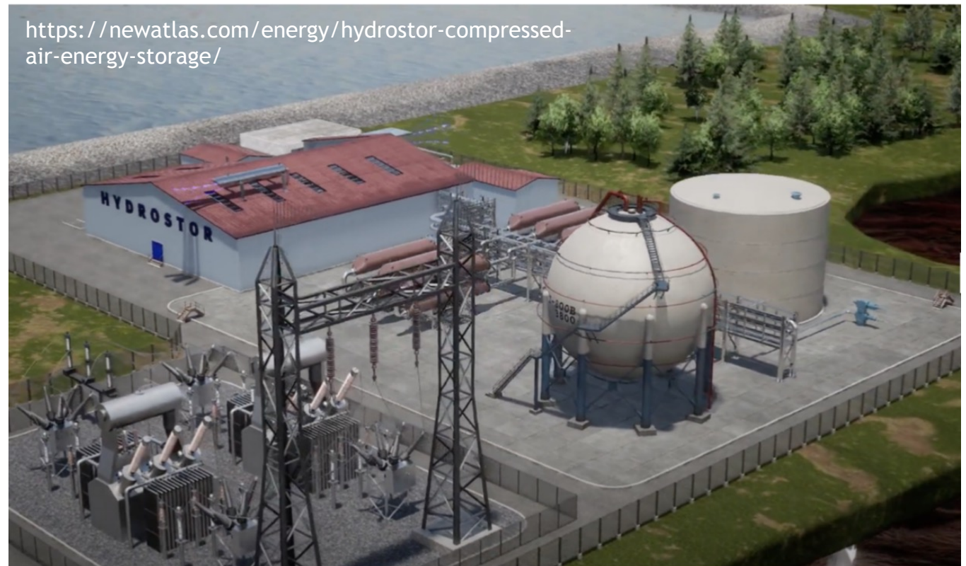
Proposed Hydrostar plant, planned to provide 500 MW, 4GWh (Rosamond, CA)
