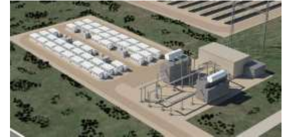
Tesla/SoCal Edison Energy Storage Station
