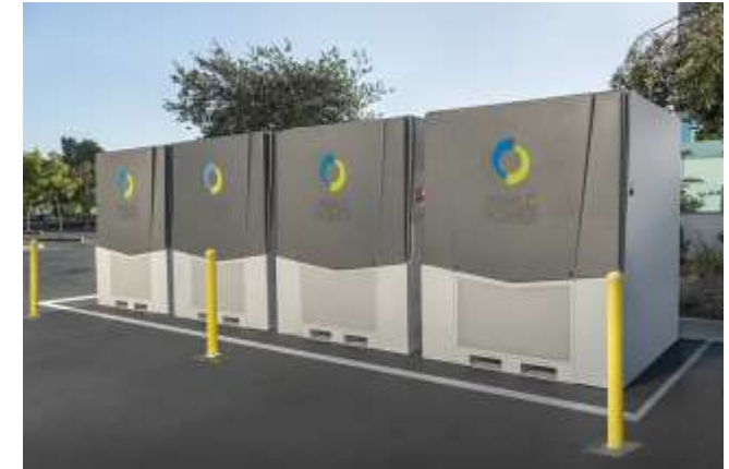
Primus Power modular Zn-Br, each unit is 25kW/125kWh
