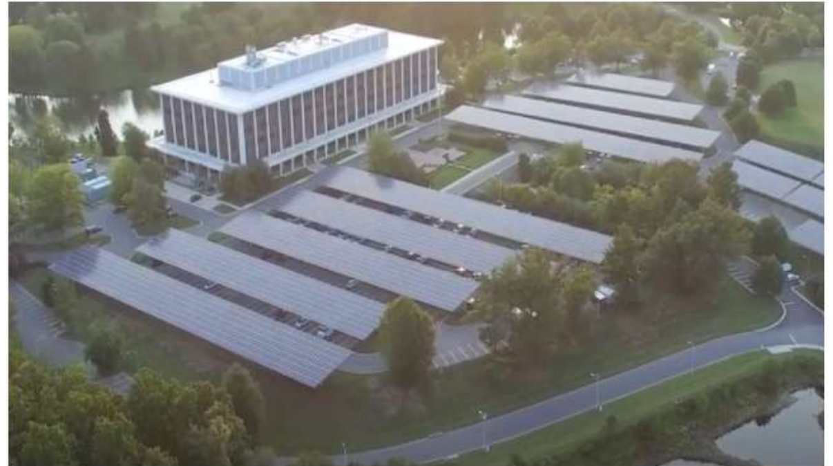
Microgrid installed at Montgomery County Public Safety Headquarters Photo Credit: Montgomery County, MD
