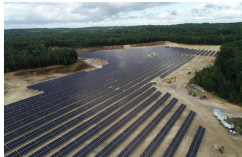
Happy Hollow Community Solar + Storage Farm
