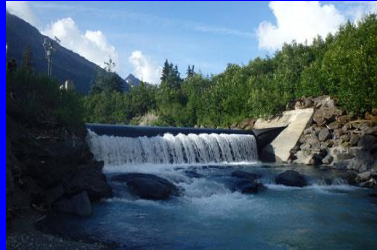
6MW Run of River Hydro Power
