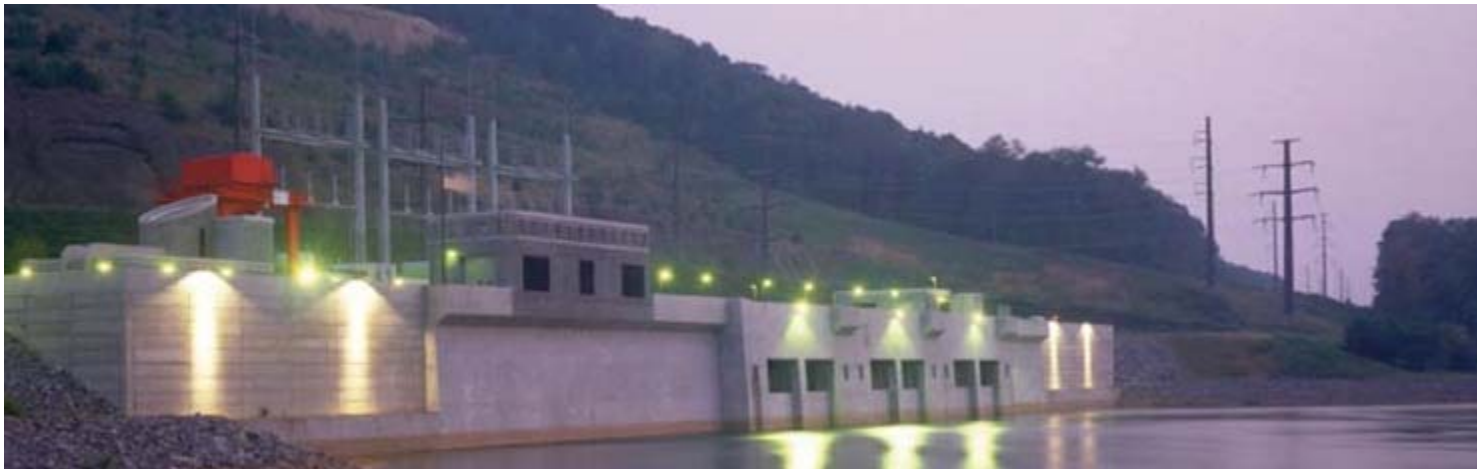
Rocky Mountain, GA commissioned 1995, 800+ MW
