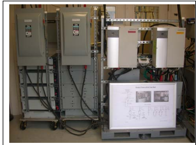
Figure 1: Grid-tied PV energy smoothing system.
