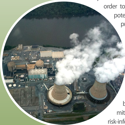
Three-mile Island Nuclear Power Plant
