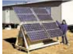
△ Energia's 600 watt stand-alone FireFly (using BP-275 modules, a Trace sine wave inverter, and Exide batteries) provides electricity to a family living on Pajarito Mesa, a colonia, or unincorporated Hispanic community. While only 5 miles from Albuquerque, New Mexico, about 150 families live without electric service. [Photo courtesy Energia Total]
