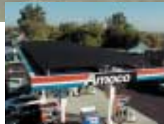
◁ This 6kW grid-connected system at a service station in Olney, Maryland, supplies 15 percent of the station's electrical needs. It is the first to use Solarex's MST43 thin film modules. [Photo courtesy Atlantic Solar]
