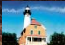
◁ Aids to navigation are some of the most popular uses for photovoltaics. Pictured here is a PV array for the Au Sable Light Station complex. The highest subarray, with the horizontal bar above it, is designed to always be above the snow level so that some solar power will be available throughout the winter. Snowfalls at the area have reached 70 inches. The horizontal bar is for protection from falling trees. The inset photo is the quaint lighthouse at Au Sable, Michigan, a registered historic site. The system was designed and installed by Currin Corporation, Midland, Michigan. [Photos courtesy Currin Corporation and Sandia National Laboratories]
