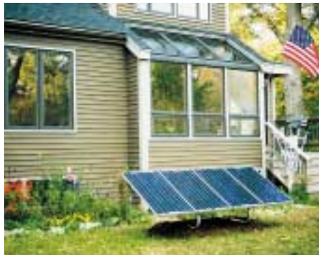
◁ Ascension Technology provided this 2kW array on a grid-connected home in the Minneapolis, Minnesota, area. The project was part of Northern States Power Company's Solar Advantage Program. [Photo courtesy Ascension Technology]
