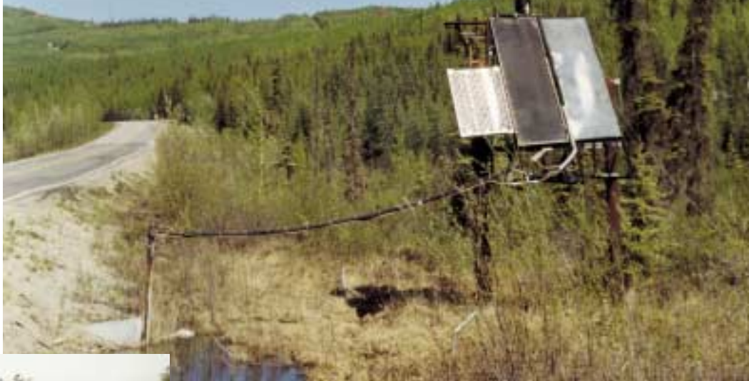
▷ A Siemens panel provides power for a public telephone where there would otherwise be none. This type of application is an excellent match for PV whether in a foreign country or in the United States. [Photo courtesy Siemens Solar]
