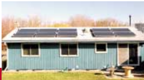
◁ Ascension Technology provided this 2kW array on a grid-connected home in the Minneapolis, Minnesota, area. The project was part of Northern States Power Company's Solar Advantage Program. [Photo courtesy Ascension Technology]
