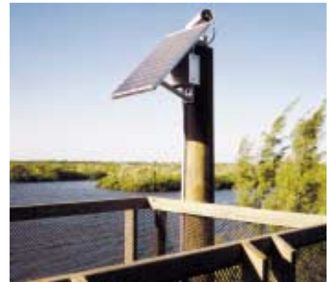
▷ A 100W Solar Electric Power assembly operates a digital camera monitoring system, which scans a major waterway for marine traffic. The system operation and location are confidential, but this type of high security system is growing popular for many applications. Similar systems operate recording devices, power alarms, and power remote video surveillance systems, to name just a few security-type applications. [Photo courtesy SEPCO™ – Solar Electric Power Company, Ltd.]
