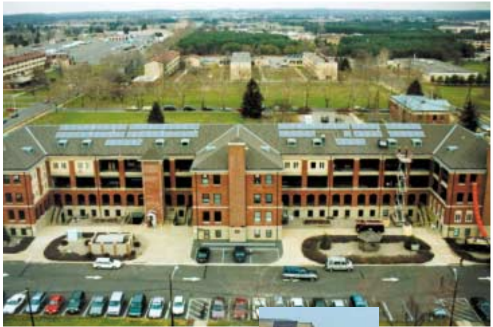
△ This 18kWp grid-connected system was installed by Ascension Technology as part of an EPA/DOE/DoD program at Ft. Dix, New Jersey for the U.S. Army. [Photo courtesy U.S. Army]
