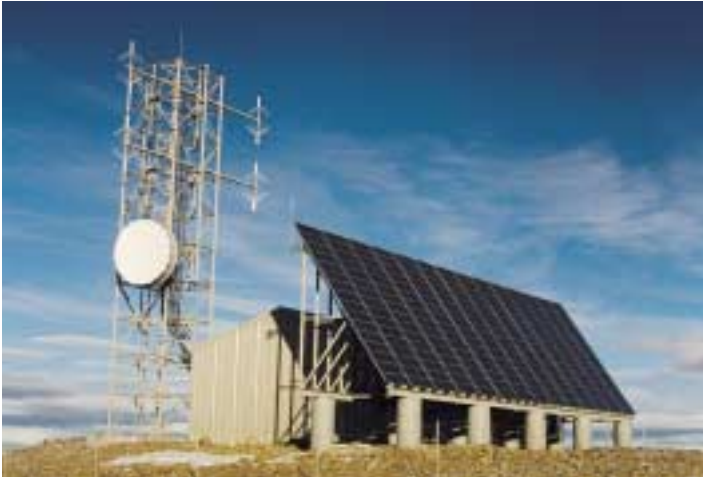
△ Northern Power Systems designed, manufactured, and installed a hybrid MicroGrid™ PV/diesel system on a 10,200' mountaintop site (Mt. Callaghan) in Central Nevada. The system serves as a master site for the Top Gun Tactical Air Combat Training System upgrade on the U.S. Navy's Fallon Range. The power system consists of an 11,872-peak watt PV array coupled with a 20kW diesel generator set. [Photo courtesy Northern Power Systems]
