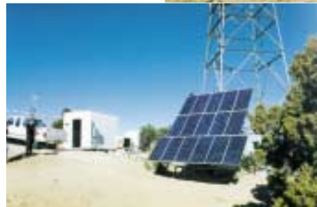
◁ Solar Depot installed this solar-powered pair-gain system. This application is well suited to PV. The twisted pairs of wire, stretching far enough that they lose their signal, benefit from the addition of a PV-powered amplifier. [Photo courtesy Solar Depot]
