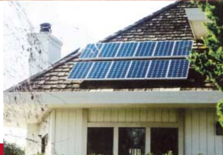
▷ A 2kW grid-tied residential rooftop system in Fairfield, California. [Photo courtesy BP Solar]
