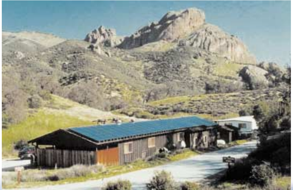
△ One of the most successful photovoltaic facility power installations has been the one at Chaparral, Pinnacles National Monument, California, for the National Park Service. A 10kW roof-mounted array (Solarex modules) provides facility power to park residences, a ranger contact station, a maintenance building, and a campground. The hybrid system (installed by Applied Power Corporation) includes a 20kW propane generator and totally eliminates the use and storage of diesel fuel in the Chaparral area. [Photo courtesy Sandia National Laboratories]
