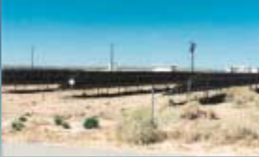
△ First Solar (formerly Solar Cells, Inc.), Toledo, Ohio, provided this 25kW de system used at the Naval Air Warfare Center, Weapons Division, China Lake, California, at a fuel cell experimentation site. NASA uses the off-grid installation for experimental purposes, indicating its interest in PV working in tandem with fuel cells. [Photo courtesy First Solar, LLC]
