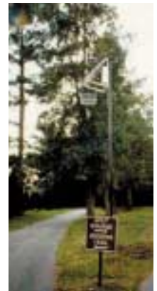
▷ PV powers lights for a jogging trail on Charleston Air Force Base, South Carolina. According to the base energy manager, he preferred solar to conventional electrical lights in order to avoid transformers and buried cables. [Photo courtesy Solar Outdoor Lighting]
