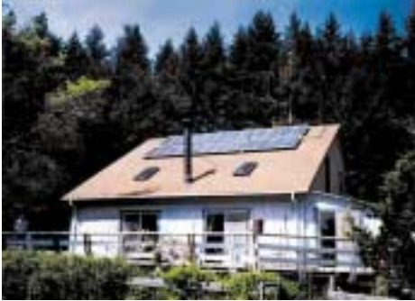
△ Bonny Doon, near Santa Cruz, California. Although this home is grid-tied, the location is remote enough that they lose power fairly often during winter storms, making a battery back-up system perfect for them. The array features 24 AstroPower 1106 V modules (1,120W ac), a Trace SW 4048 inverter, and four flooded Trojan batteries. The installation, provided by Pacific Solar Company of Redwood City, California, provides most, but not all, of their electrical needs. [Photo courtesy Pacific Solar Company]
