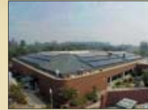
△ The Western Area Power Authority building in Folsom, California, features 12kW Solarex, 12kW EPV, and Trace inverters on its line-tied PV system designed and installed by Solar Electrical Systems, Thousand Oaks, California. [Photo courtesy Solar Electrical Systems]
