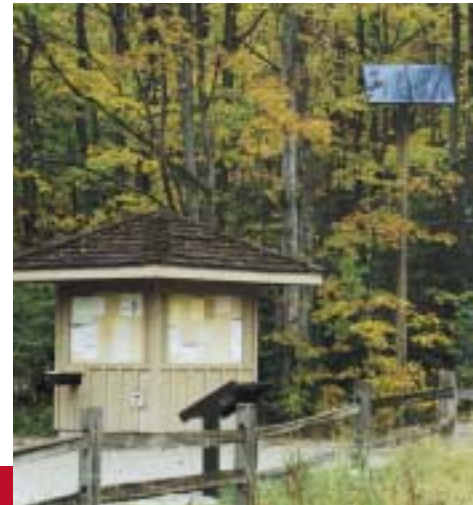
▷ A 24V solar-powered water pumping system is located at the picnic area/trailhead at Pictured Rocks National Lakeshore, Grand Marais, Michigan. Called the Log Slide Pumphouse, the installation was designed by Currin Corporation and is contained in the kiosk structure that also serves as an information station and storage building. [Photo courtesy National Park Service]
