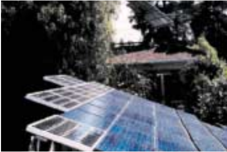
△ Ed Begley, Jr., actor and environmentalist, admits his off-grid solar-powered home in the heart of Los Angeles is a sizeable investment, but he wouldn't want to live any other way. His system is comprised of 100 60-watt panels. He has the requisite large battery bank and sinewave inverter in his garage—where he also keeps his PV-charged electric car. [Photo courtesy Ed Begley, Jr.]
