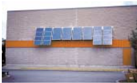
◁ BJ's Wholesalers in North Dartmouth, Massachusetts, serves as host to Sun Power Electric's first power plant. Following utility deregulation in Massachusetts, environmentally conscious electricity consumers' needs are being met through this 'green electric' product. There are actually three PV systems on BJ's. Two are wall mounted and one is roof mounted using special clips on a standing seam roof. The PV consists of 4 SunSine AC modules from Ascension Technology, 4 Evergreen Solar AC modules, and a 12kW ASE Americas system. [Photo courtesy ASE Americas]
