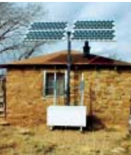
◁ The large remote Navajo Nation in Arizona and New Mexico is the ideal setting for photovoltaic power systems. This home is in the Whitehorse Chapter of the Navajo Nation, where 22 identical systems were installed by AAA Solar. All systems include four Siemens 100W modules on a pole mount, eight Exide E-3600 220 AH deep-cycle batteries, and a Trace DR series 2400W inverter. Enough power is produced for lighting, some small appliances, and a very efficient small refrigerator. [Photo courtesy AAA Solar]
