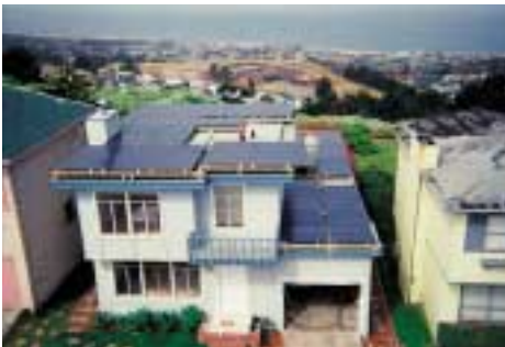
▽ This roof-mounted 10kW system powers a single residence overlooking the Pacific Ocean. Concorde sealed batteries and two Trace SW5548 inverters accompany 96 AstroPower 1206 modules, designed and installed by Pacific Solar Company. [Photo courtesy Pacific Solar Company]
