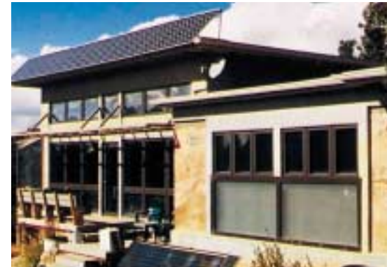
▽ In the Williamson Valley of Arizona, 18 Siemens Solar panels run along the roof edge (smaller panel is for hot water) of this off-grid home. Designed and installed by EV Solar Products, Chino Valley, Arizona; products provided by Hitney Solar. The installation uses a Trace inverter and Trojan batteries, together providing a 1.35kW array for the residence. [Photo courtesy EV Solar Products]
