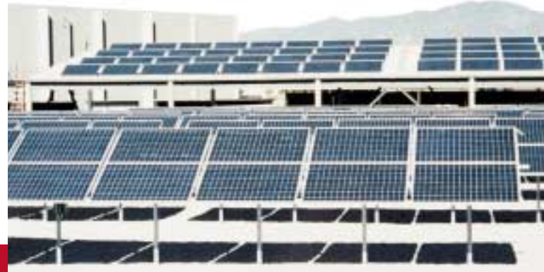
▽ A 120kW array of ASE Americas 300-DG modules was installed by Applied Power Corporation at the Bentley Mills carpet factory in Southern California. APC (Lacey, Washington) also designed the installation, which is one of the largest industrial solar installations in the United States. Bentley Mills is a subsidiary of the Interface Group, a global provider of flooring products with a philosophy of sustainable manufacturing. [Photo courtesy ASE Americas, Inc.]
