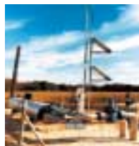
△ A Hutton Communications installation for a natural gas utility provides flow monitoring for oil pipelines and wells in Oklahoma and elsewhere. This type of remote telemetry is an ideal application for photovoltaics. [Photo courtesy Hutton Communications]
