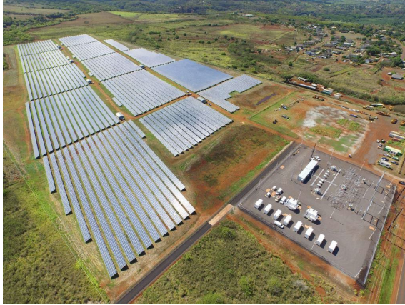
Saft 6 MW / 4.2 MWh ESS Kauai - Grid Stability
