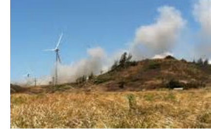
2012 Battery Room Fire at Kahuku Wind-Energy Storage Farm
