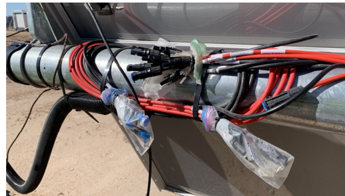
Open connector, not fully engaged.
