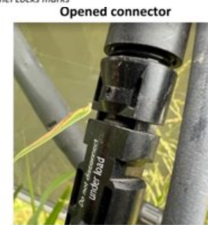
Open connector, not fully engaged.
