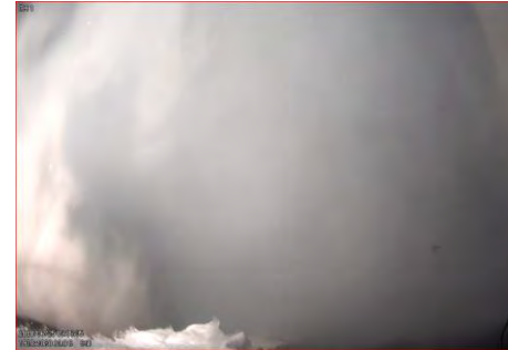
Novec 1230 discharge [TR + 00:00:58]
