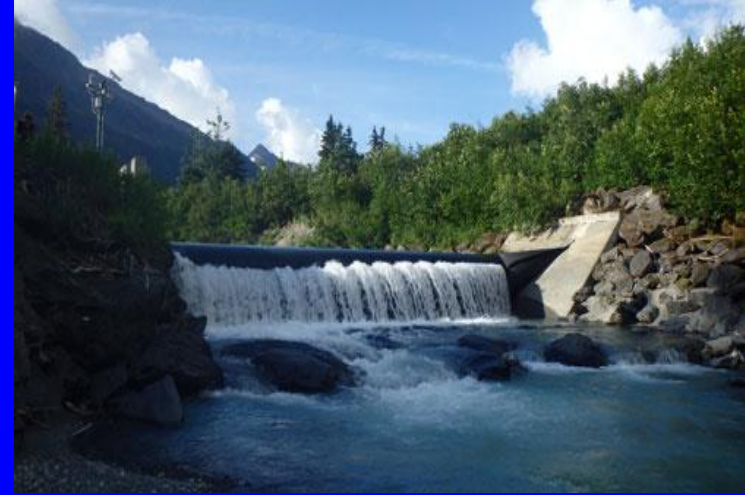
6MW Run of River Hydro Power
