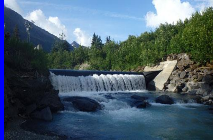
6MW Run of River Hydro Power
