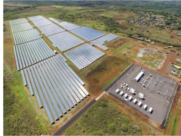
Saft 6 MW / 4.2 MWh ESS Kauai - Grid Stability
