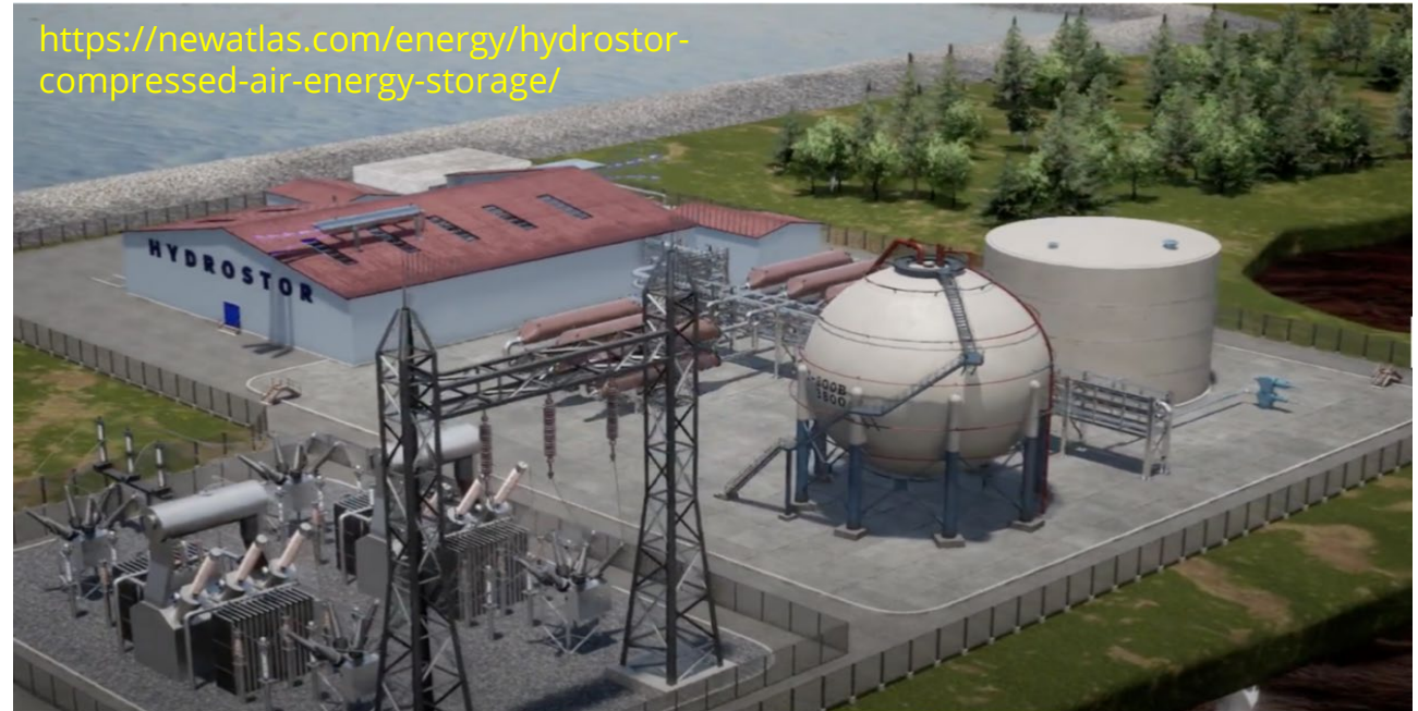
Proposed Hydrostar plant, planned to provide 500 MW, 4GWh, (Rosamond, CA)
