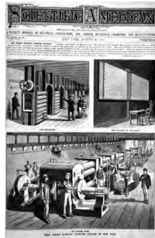
Edison's first commercial plant, Pearl St., NY 1882
