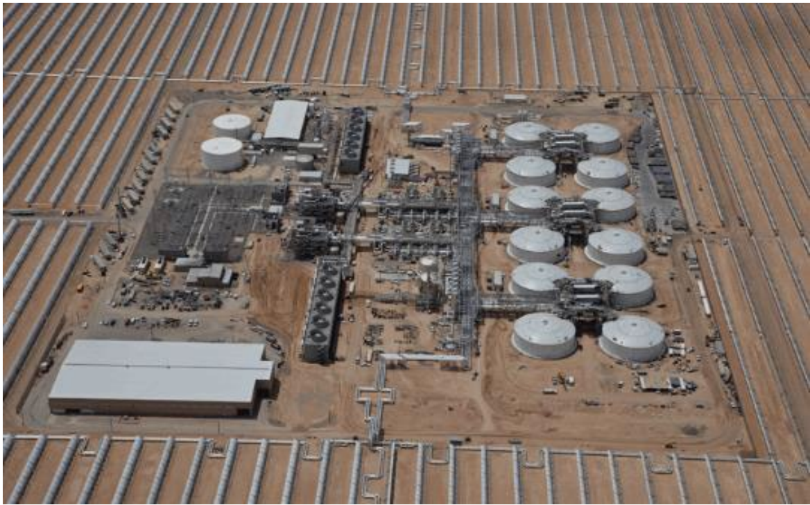
Solana Parabolic Trough Plant, AZ (280 MW e with 6 hrs storage (1.5 GWh e ))
