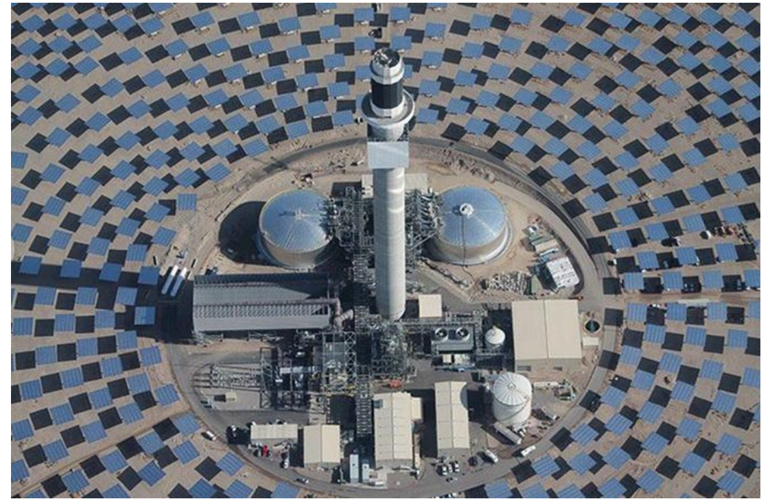
Crescent Dunes Solar Tower, NV (110 MW e with 10 hrs storage (1.1 GWh e ))
