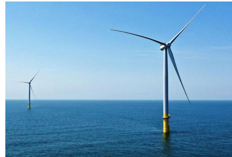
Dominion Energy CVOW Site
