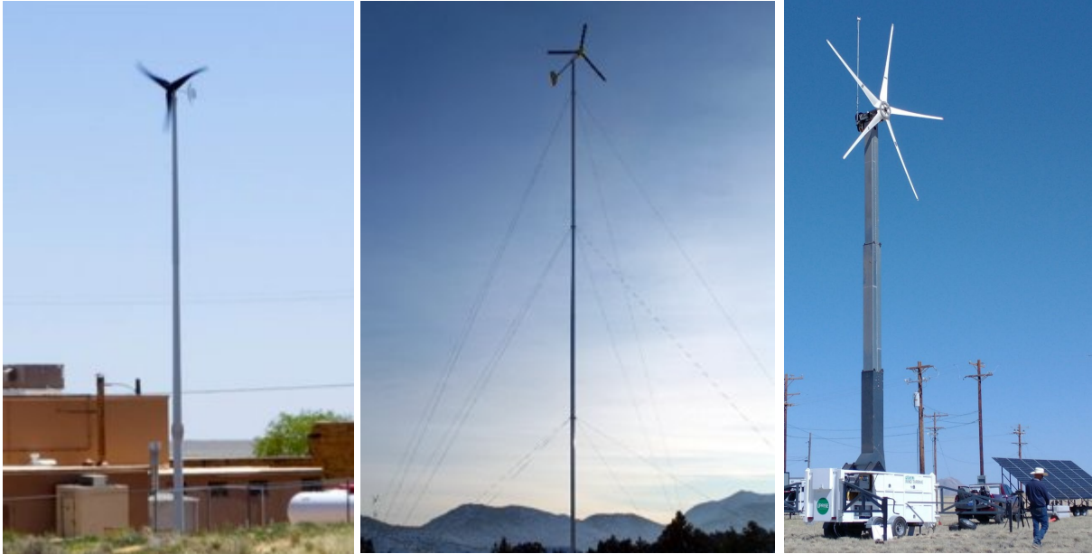
Figure 6. Single-piece, monopole tower (left, Pika Energy turbine, NREL PIX 31470), segmented, guyed tower (center, Bergy Windpower turbine, NREL PIX 16742), and telescoping tower (Uprise Energy turbine, Idaho National Lab)
