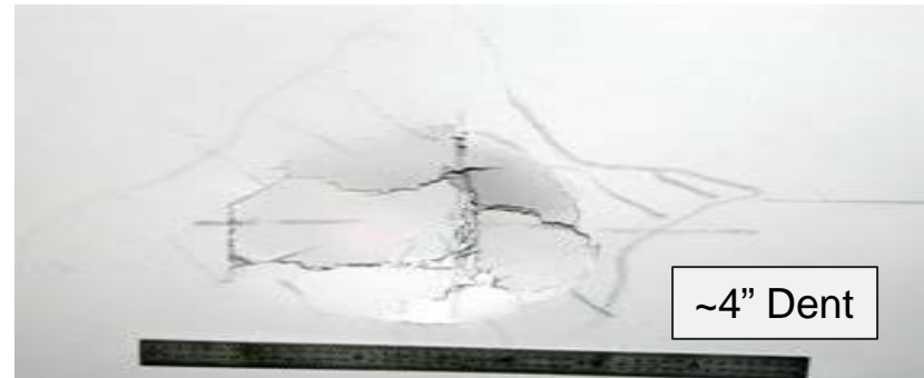
Exterior Skin Damage
