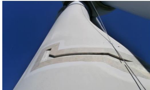
Extensive repair is made
