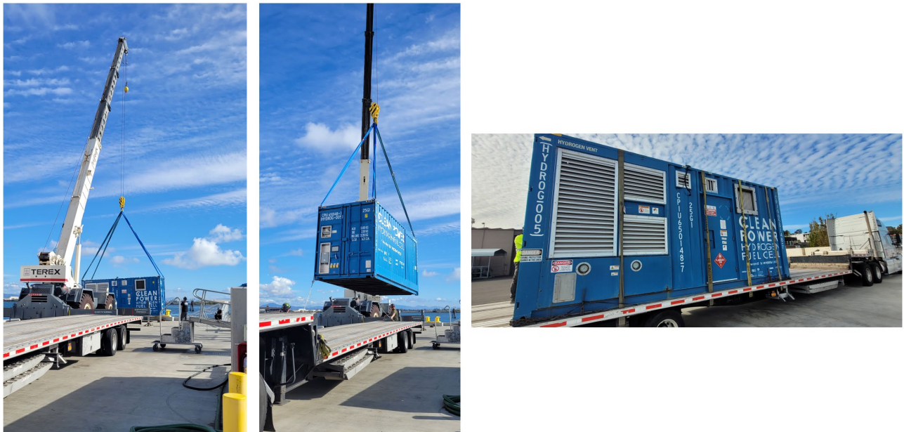
Figure 31. (L) Craning the MarFC unit off the SIO Pier; (M) Craning the MarFC onto the flatbed truck and (R) The MarFC secured to the flatbed truck ready for shipment to Minnesota.
