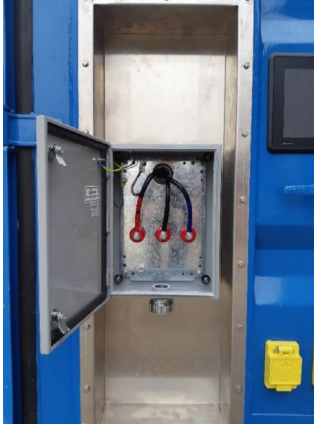
Figure 13. New recessed connector panel/box mounted on the MarFC unit for use at SIO.
