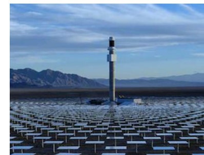
Crescent Dunes, molten salt, 110 MW e , NV, 2015
