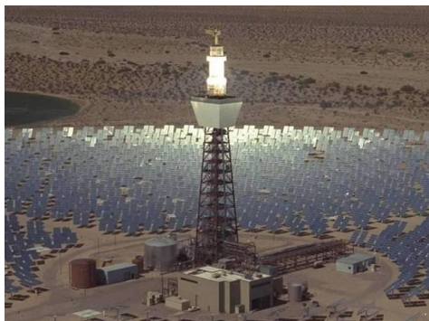
Solar One and Solar Two 10 MW e Daggett, CA 1980's - 1990's
