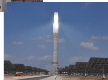
Gemasolar, molten salt, 19 MW e , Spain, 2011
