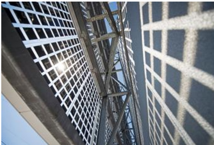
Figure 4: SWCT-CSEM Façade -Semi-transparent facade of the renovated CSEM building in Neuchâtel, Switzerland, which comprises bifacial SHJ cells interconnected by SWCT™.
