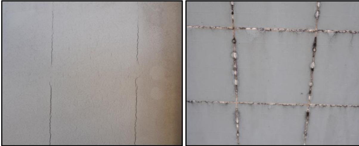
Figure 10: PA cracks. Longitudinal and squared cracks of PV modules with PA backsheets [7].
