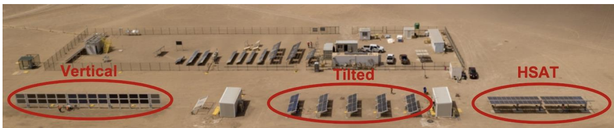
Figure 74: ATAMOSTEC Bifacial PV testing platform, Antofagasta, Chile
