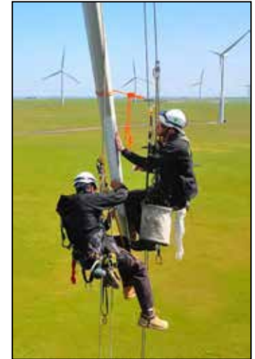
Scarfed Blade Repair Process
