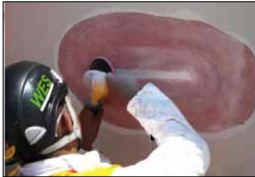
Scarfed Blade Repair Process
