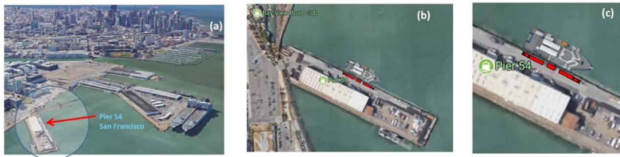
Figure 30: Location of Pier 54, San Francisco CA. (a) General Pier 54 location relative to the City of San Francisco; (b) general view of Pier 54 with the Zero-V docked and (c) close-up view of the Zero-V docked at Pier 54 along with two LH 2 trailers and refueling stanchion show in red. The refueling stanchion is notional only. The relative sizes of the Zero-V, LH 2 trailers and dock are properly rendered. Satellite images are courtesy of Google Maps.
