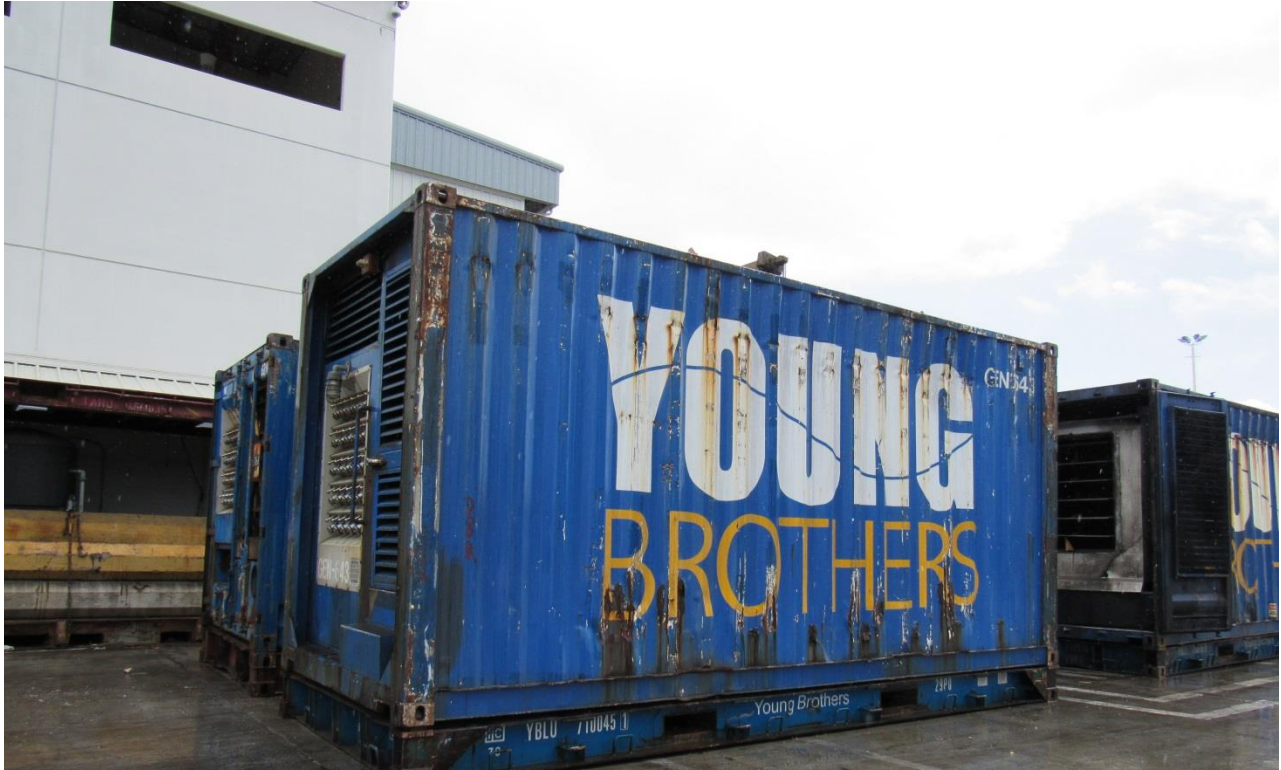
Figure 2. Typical diesel generator sets used to provide electrical power to refrigerated shipping containers at dock side and in transit between islands.
