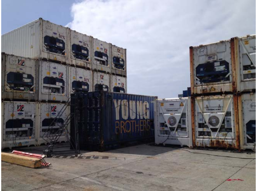
Figure 7: Diesel generator (blue) powering reefers (white) on the dock at Young Brothers' Honolulu facility.
