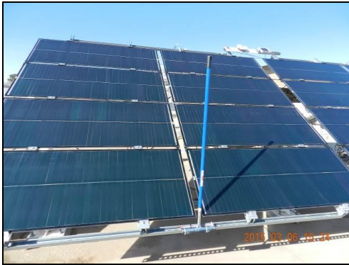
Fig. 10. Picture of the pole shading test setup.
