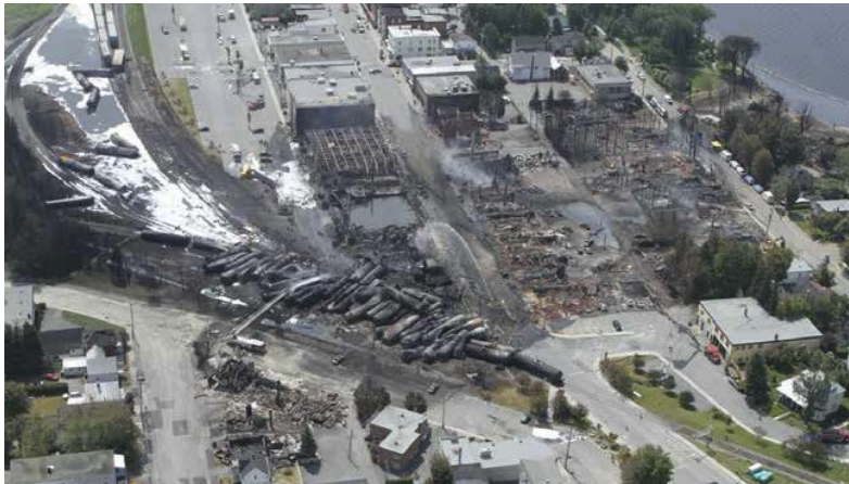
Figure 7-2. Post-accident Site at Lac-Mégantic, Quebec.
