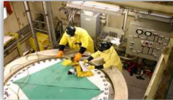
Lid Installation of a TN-32 Cask
