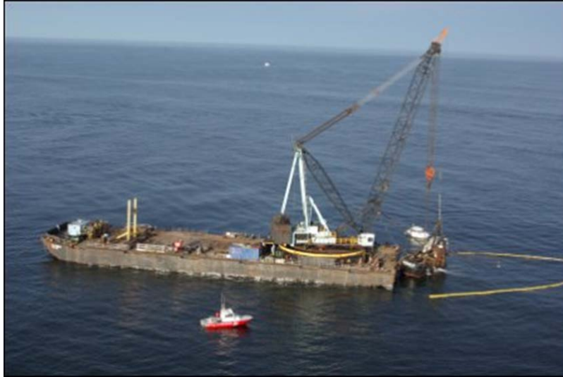
Figure 6-35. 400-foot crane barge with 400-tonne crane lift capacity.
