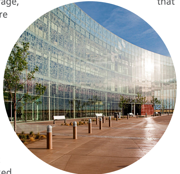
The Mesa Del Sol Aperture Center is located in Albuquerque, New Mexico. Photo courtesy of Jon Anderson Architecture.
