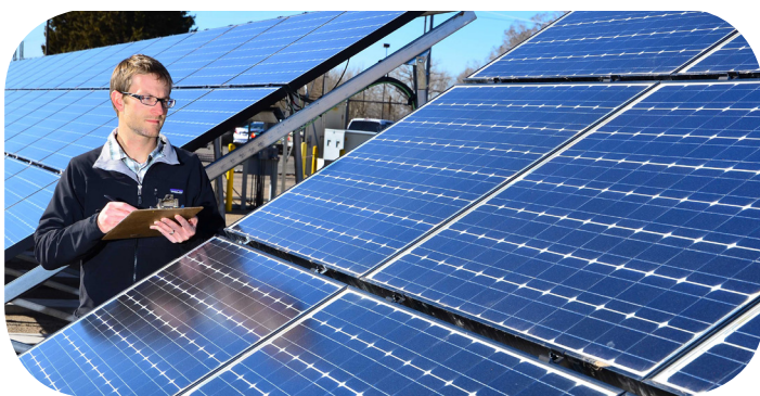
Sandia researcher Geoff Klise originally worked with Solar Power Electric™ (now Energy Sense Finance, LLC) to develop a tool that can be used to appraise photovoltaic installations on homes and businesses. (Photo by Randy Montoya)
