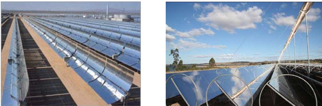
Figure 5. Parabolic trough (left) and linear Fresnel (right) collector systems (photos from [http://en.wikipedia.org/wiki/Solar\\_thermal\\_energy](http://en.wikipedia.org/wiki/Solar_thermal_energy)).
