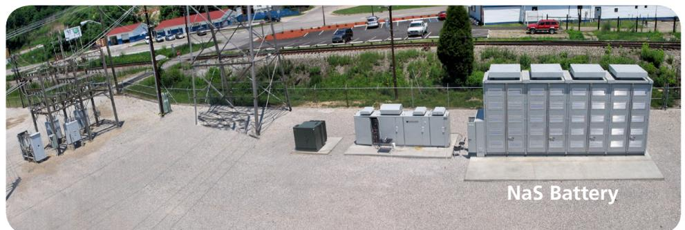
*This Sandia-led DOE Office of Electricity demonstration project proved the effectiveness of sodium-sulfur batteries in peak shaving and capital deferment.*
