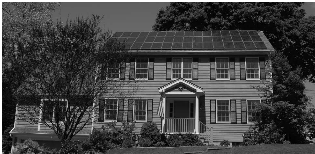
Figure 1 Photo of Array on Rooftop
