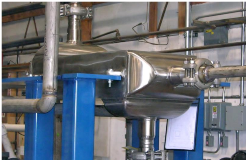
Figure 2-8. S-CO 2 high-temperature PCHE recuperator.
