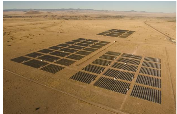
Fig. 2. TEP Springerville Photovoltaic Generating Facility.
