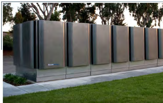
Figure 8: Bloom Energy ES-5700 solid oxide fuel cells, each producing power at 210 kW each. Photo from Reference [43].
