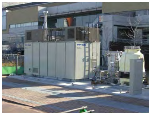
Figure 11: Fuji Electric 105 kW, Model FP-100i PAFC. Photo from Reference [47].
